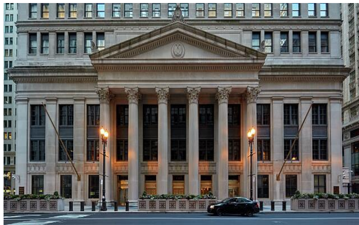
Fig. 1. Federal reserve bank building [15]
