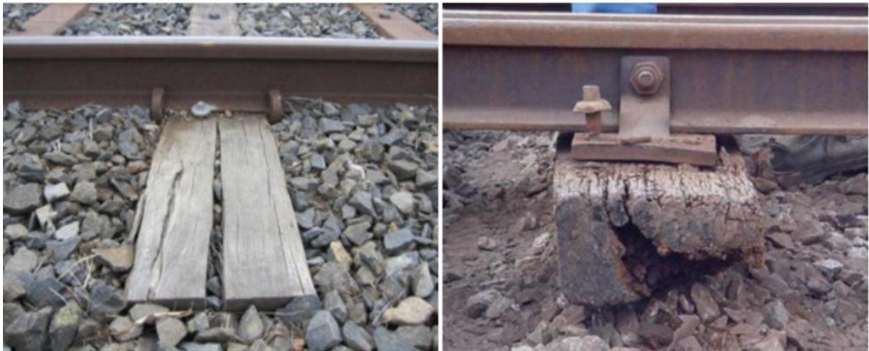
Fig. 1. Aged timber sleeper [6]
