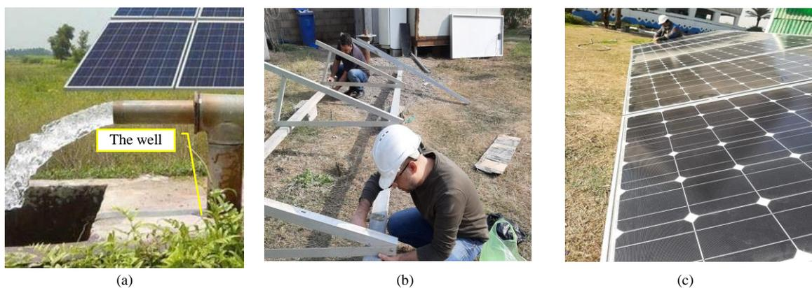
Fig. 5. Photos for the well under study; a) the well, b) the PV array structure, and c) the PV array
